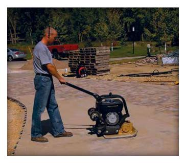
Figure 11. Vibrating sand into the joints.
