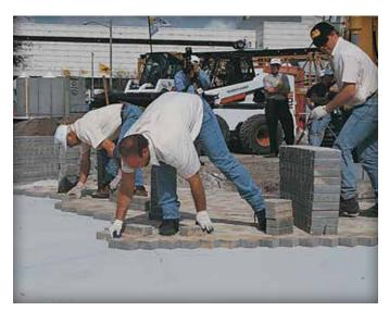
Figure 7. Placing the concrete pavers.
