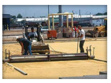
final base surface elevations should not exceed  $\pm \frac{3}{8}$  in. ( $\pm$  10 mm) when tested with a 10 ft. (3 m) straightedge.
