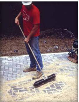
Figure 10. Spreading the joint sand.
