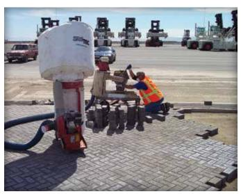
Figure 8. Saw cutting pavers.
