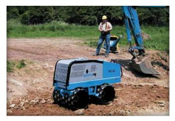
Figure 2. Compacting the soil subgrade.
